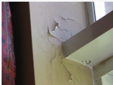
A home inspection revealed that all of the windows were installed wrong on this 3-year-old multi-million dollar home.
